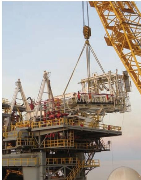
Left EDrill-1 Rigging Up September 2014 - Most landed and secured atop Drill Floor
